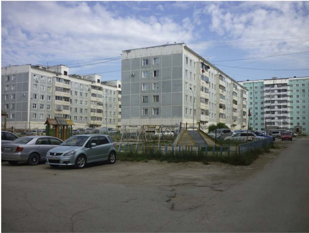
Fig. 2. Large-panel buildings of the 112 series in “Mikroraion 202” area, constructed in the late 1980s. Photograph: J. Otto Habeck.
