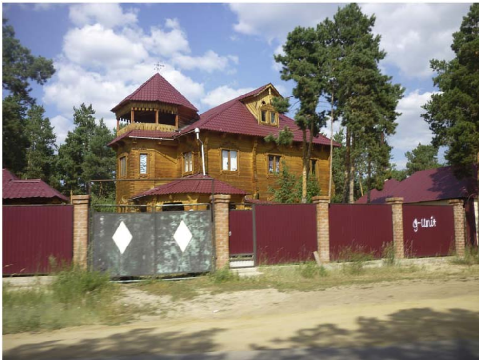
Fig. 4. A newly-built wooden villa at Sergeliakhskoe shosse, locally known to be one of the most prestigious areas of Yakutsk. Photograph: J. Otto Habeck.
