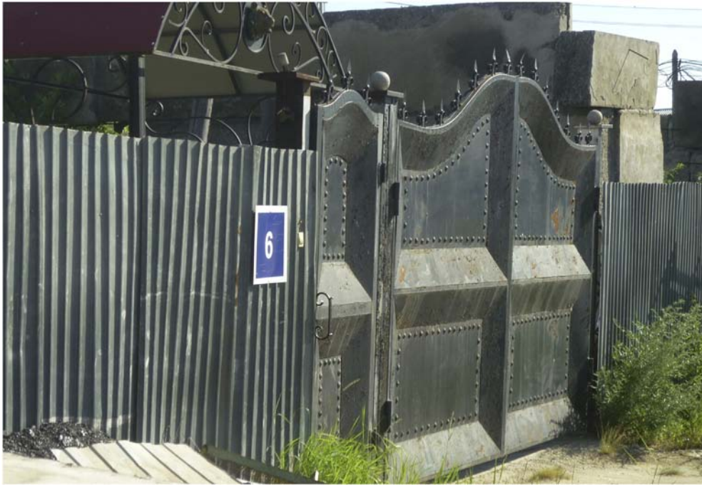
Fig. 7. A proflist fence with a self-made gate, featuring metal plates and wrought iron (the plot is located in the area of Zalog). (For interpretation of the references to colour in this figure, the reader is referred to the web version of this article.) Photograph: J. Otto Habeck.
